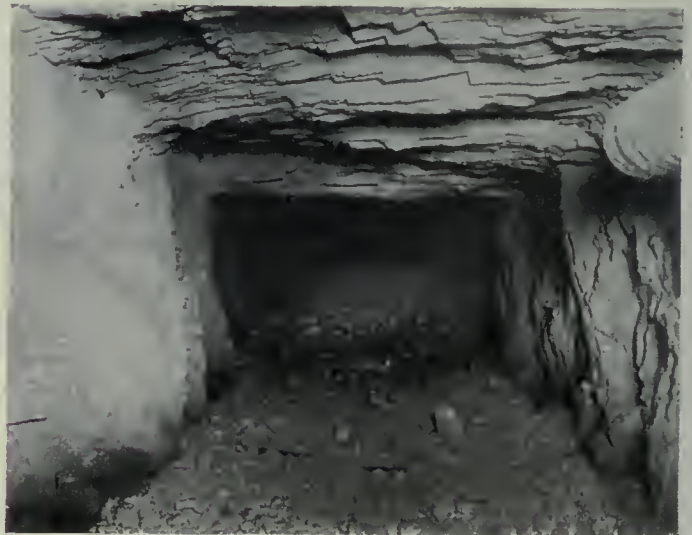
Final connection of the Pioneer Tunnel—Looking west
